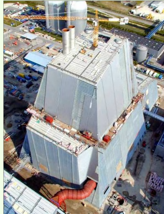
The 570MW Avedøre-2 power plant in Denmark, during construction
